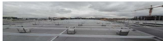
Purlin to support solar module
