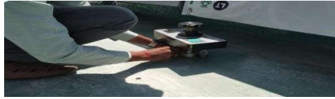
Pull out test to check bond adhesion.
