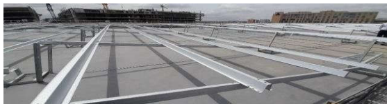
Purlin to support solar module
