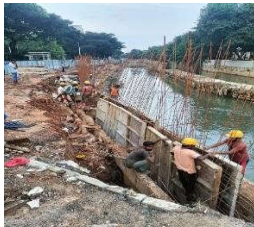
Wall reinforcement & shuttering work in progress.
