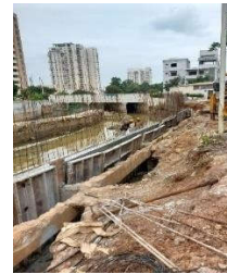
Wall reinforcement work in progress.
